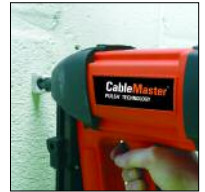
3. Attach clip to pin guide. Depress and fire tool.
